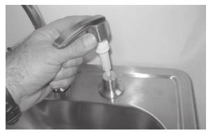
Note: You can add liquid soap to the dispenser by pouring it directly into the dispenser base after the bottle has been attached. 9
