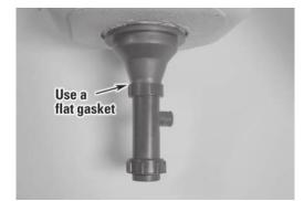
7. Attach trap (6) to drain.
