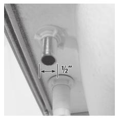
Note: An adaptor is not included with your sink. You will need to provide one for the size of your water line connection.
